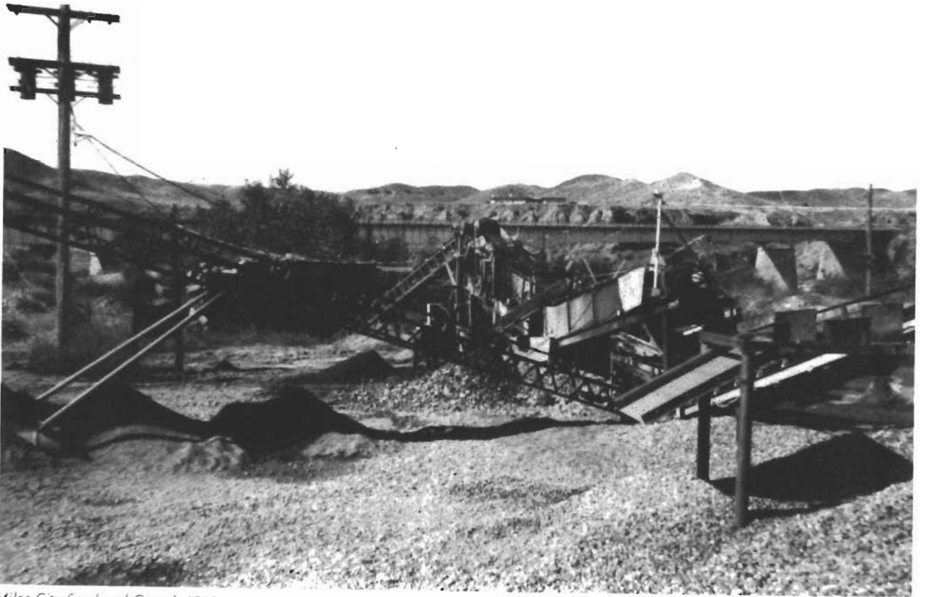
Miles City Sand and Gravel, 1962.
